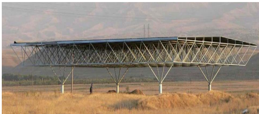
6. View of the excavation III covered with a shelter
